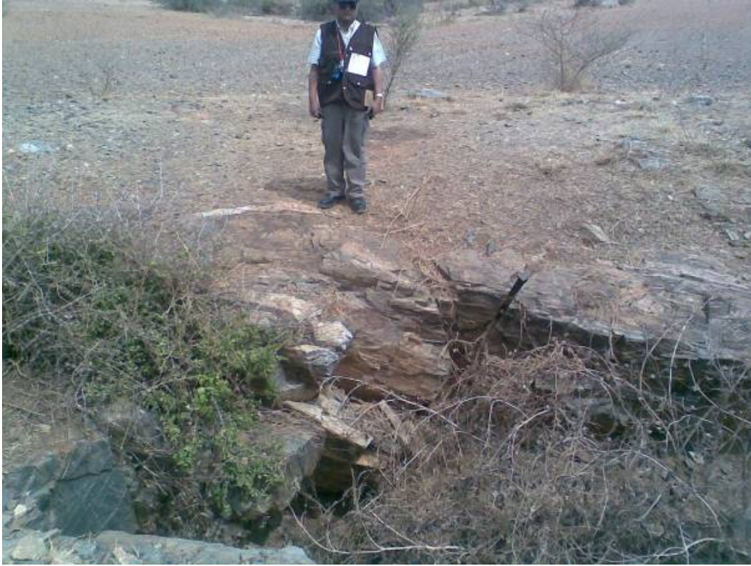
Photo 1 - Trench at Chikahonnakuni cut on quartz vein
